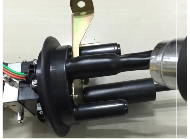
8. Sealing the shrinkable sleeve by hot-air blower
