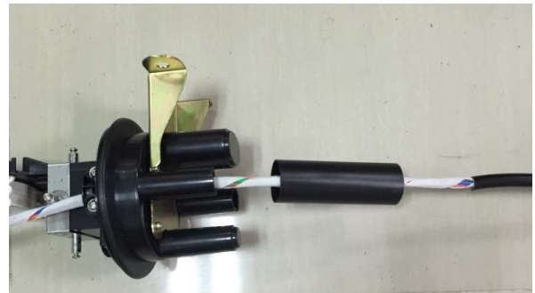
4. Put the cable through shrinkable sleeve and closure box
