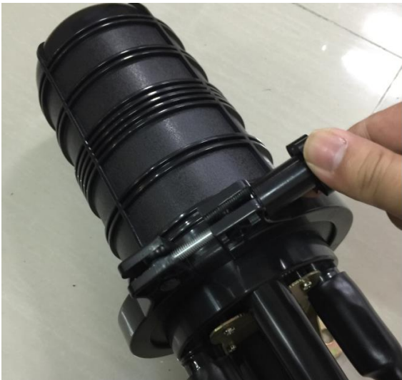
9. Put on the splice tray cover, rotate the hoop and compress it .
